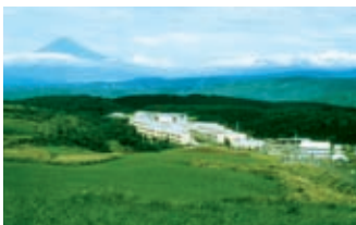
The Nakaizu Rehabilitation Center
